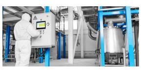
Controllers are the local control center and data hub of integrated gas detection systems. They turn the data from transmitters into actions. In turn, controllers allow the collected information to be further stored or evaluated by a higher order processing or data center. GfG offers a wide range of controllers for various applications.
